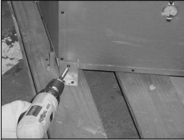
Figure 4.11 Removing Shipping Brackets
